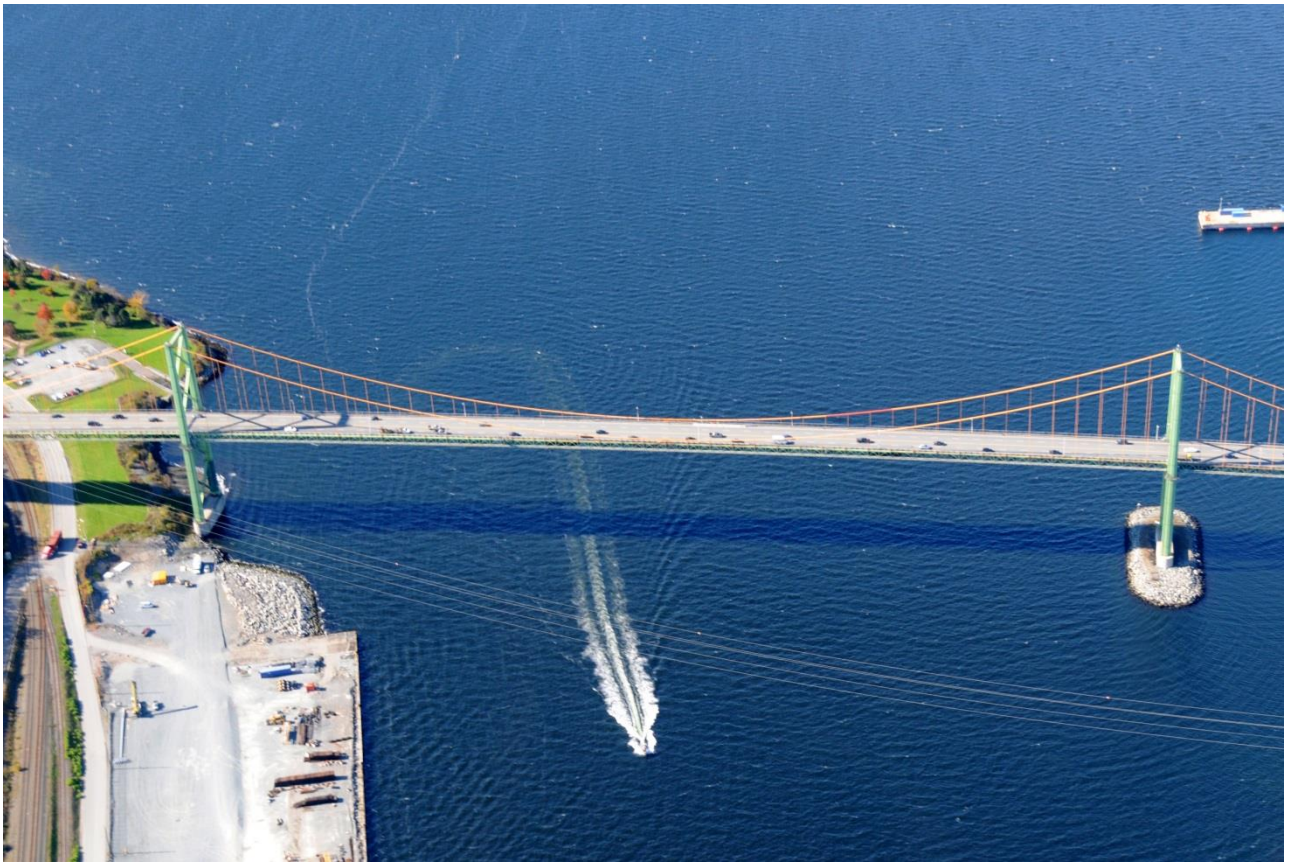
Photo: A. Murray MacKay Bridge
